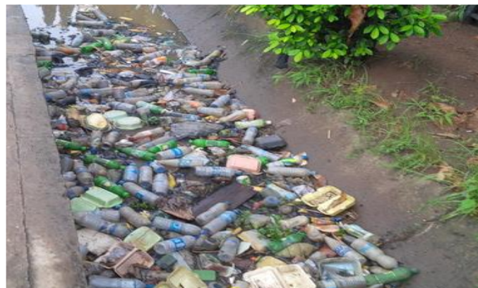
Plate 5. Blockage of Drainage - Poor waste management at Ijoka Area, Akure.
