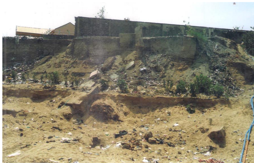
Plate 3. Foundation under threat along the riverbank of Yedzeram.
