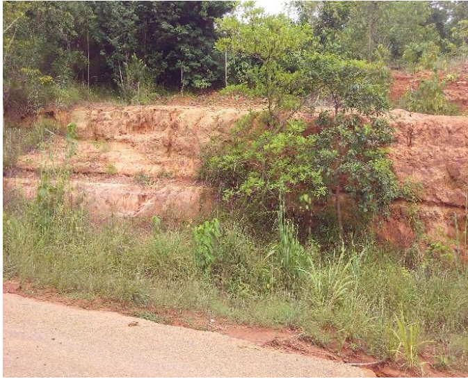
Plate 1. Exposed soil unit along Iboropa – Ise Highway.
