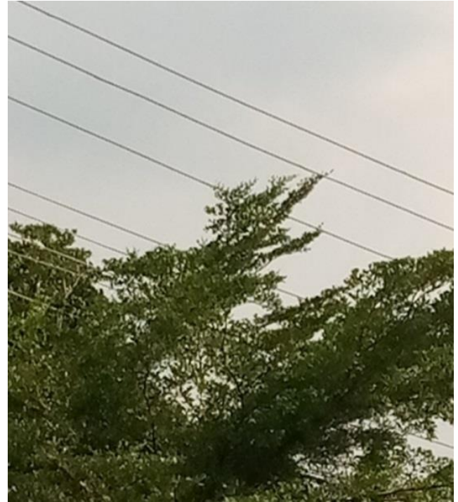
Figure 5. Secondary distribution line overgrown with trees.
