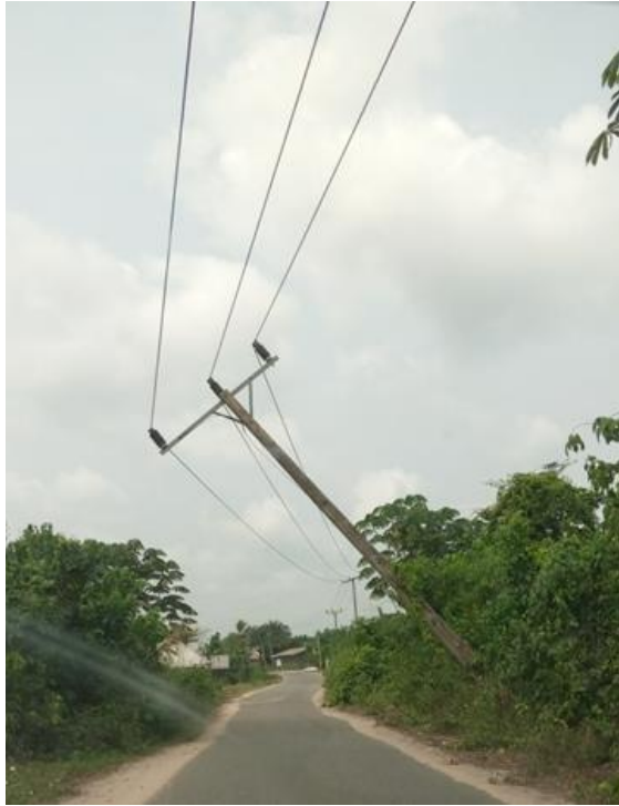
Figure 6. A slanting utility pole at Owhe community.
