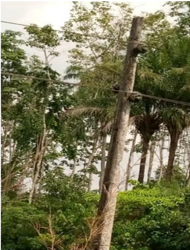
Figure 2. Insulator attached directly to the utility pole at Oleh Community.
