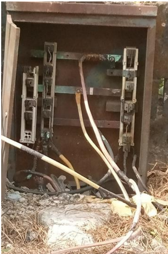
Figure 7. A transformer feeder pillar.
